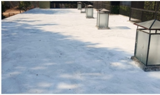
Application of Calcium Carbonate on terrace of night holding rooms to avoid sunlight absorption
